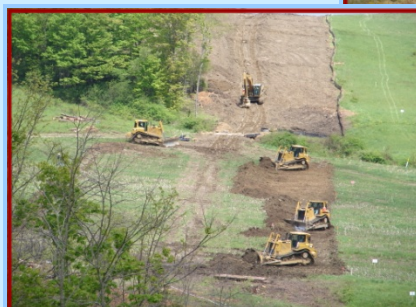
Topsoil Segregation
